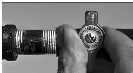
Figure 50 - Gas valve in “off” position.
