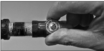
Figure 32 - Gas valve in "on" position
