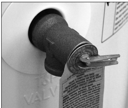
Figure 25 - Temperature and Pressure Relief Valve
