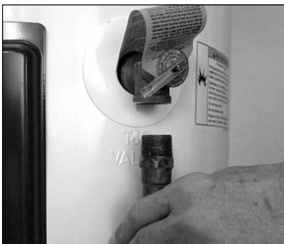
Removing the T&P Relief Valve discharge pipe.
