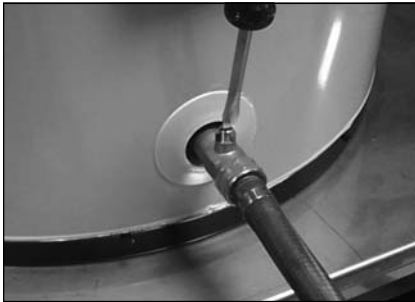
Draining the old water heater.
