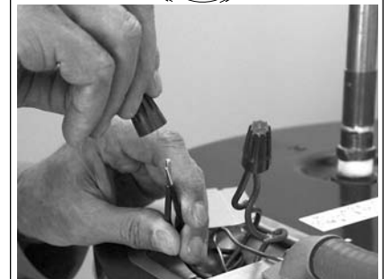
Connecting the electrical wires.
