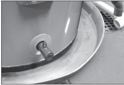
Figure 6 - A suitable drain pan piped to an adequate drain can help protect flooring from leaks and drips.
