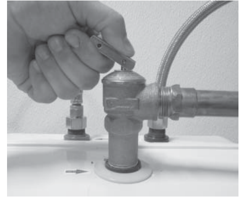
Figure 31 - T&P Relief Valve
