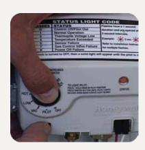
Set the temperature to the desired setting. We recommend a maximum temperature setting of HOT (120°F) to reduce the risk of scalding. See the water heater's labels for important safety information.
