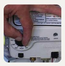
1 flash every 3 seconds means the pilot is lit and the gas valve is working normally.
