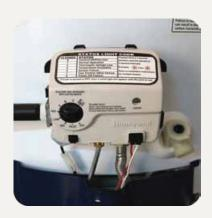
Turn the control knob to pilot and press the knob in fully. Hold the knob in and click the ignitor about once a second until the status light begins to blink. Because there is air in the gas line, it may take up to 90 seconds before the red status light begins to blink. The red status light will blink once every 3 seconds when the water heater is operating normally. Once the red status light is blinking, release the knob.
