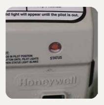
A solid red status light means the water heater is shutting down. Turn the gas control valve OFF and wait 10 minutes before attempting to relight the pilot.
