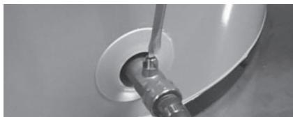
Figure 29 - Drain Valve
