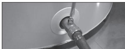
Figure 38 - Drain Valve
