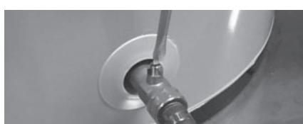
Figure 29 - Drain Valve
