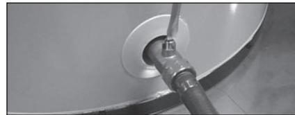
Figure 38 - Drain Valve
